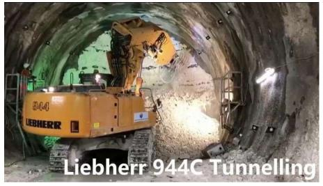
Tunnel construction is one of the toughest operating environments for an excavator to be used in. The operation of a tunnel excavator becomes efficient when the machine, despite the harsh conditions, can cut out the required tunnel profile as rapidly as possible but in economical fashion.
